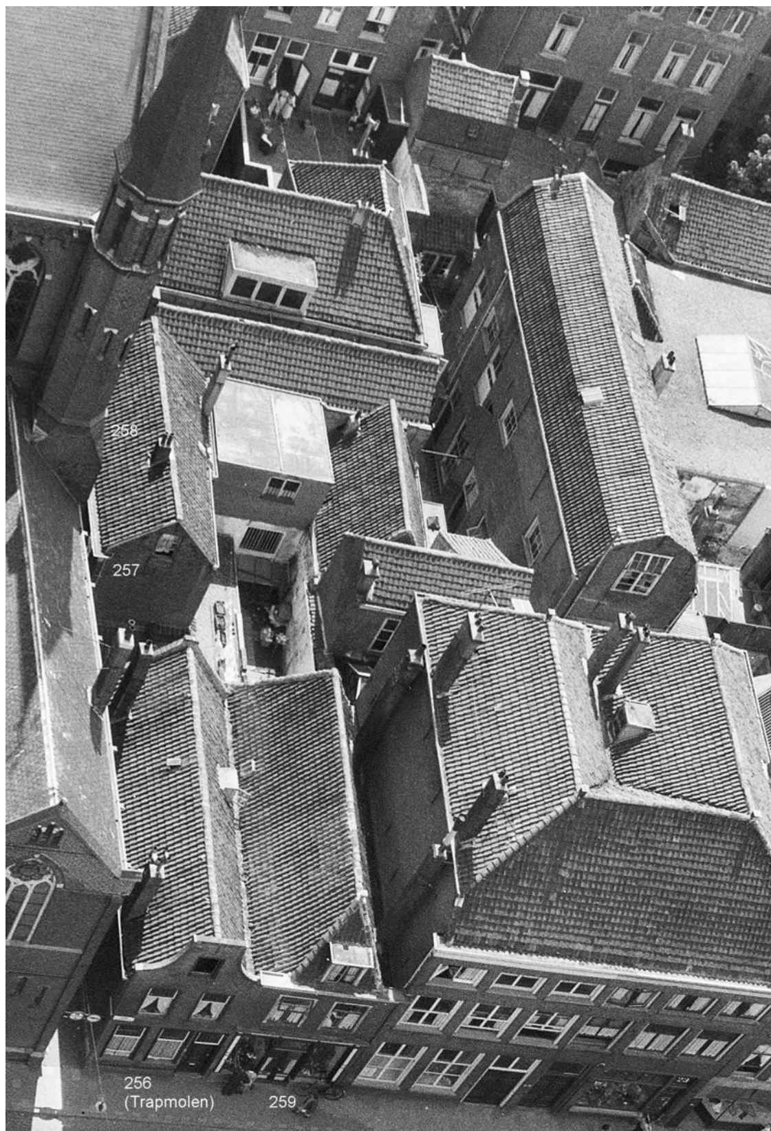
Figure 6: Oude Langendijk 25 from above (with plot numbers 256-259 from Kadastrale Minuut 1832 inserted). From: Beeldbank cultureel erfgoed, no. 68.559, photo by G.Th. Delemarre, 1962.
